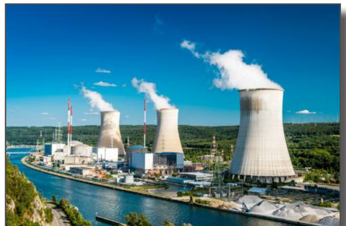
Cooling water control for power plants
